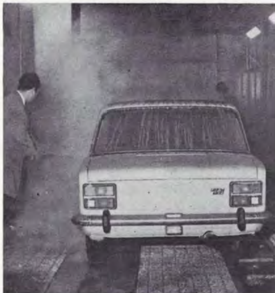
IN . . . the cars are taken from the recovery area and put through a steam spray to take off the protective layer of wax . . .
